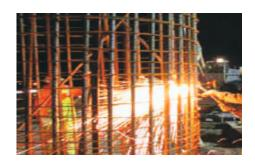
The welding performance is an important indicator of TMT bar. After welding, the microstructure and properties of the weld and heat affected area will change and become weak point of the bar. The amount of carbon content in steel has been a major deciding factor and an excess of carbon content threatens, its property of weldability. Simhadri TMT steel bar with low carbon content has In-built ability to resist loss of strength at high temperature, can be butt welded & lap- welded.
